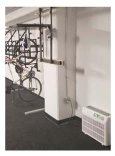
KBS has installed V-Pac HVAC units in smaller spaces served by hard-toaccess ductwork. These units are utilized for small congregation areas, like bike rooms or vestibules.
